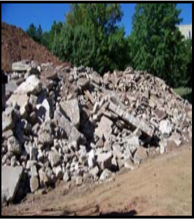
Concrete being stored in a pile
