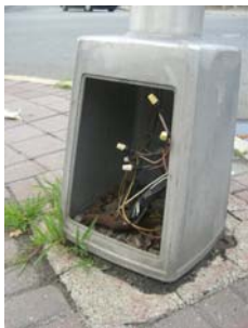
Broken/ Open Traffic Boxes
