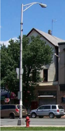
Cobra Headlight along Parcel A
