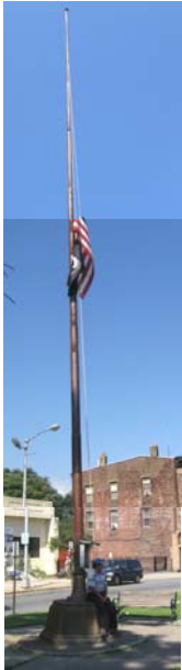
Rusted flagpole on Parcel A
