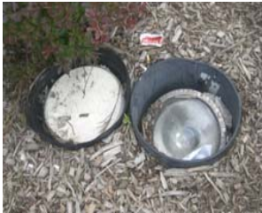
Broken Flood Lights
