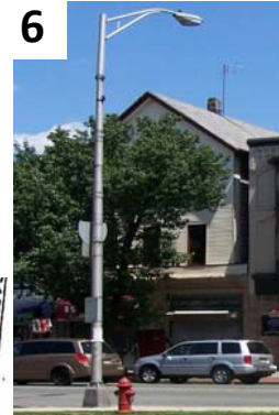
6 Cobra Street lights
